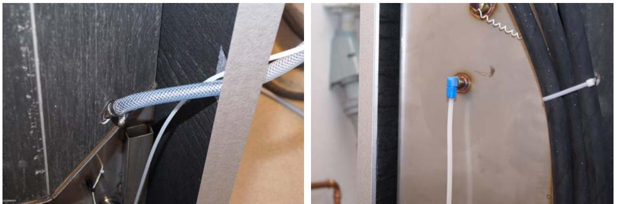
Figure 7: Detergent and rinse aid connections.
